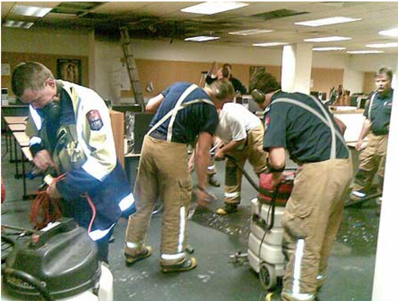
Fire Service staff clean up the damaged laboratory earlier today.
