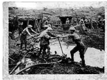
The Western Front 1917: Trying to keep dry and prevent the low-lying trenches from flooding was a constant struggle. Soldiers pumping water away from the trenches. Joan Miskimmin??.
