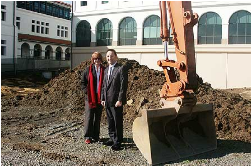
Auckland campus head librarian Valerie Cohen and Deputy Vice-Chancellor (Auckland and International) Professor John Raine at the site of the new library building with the current library in the background.
