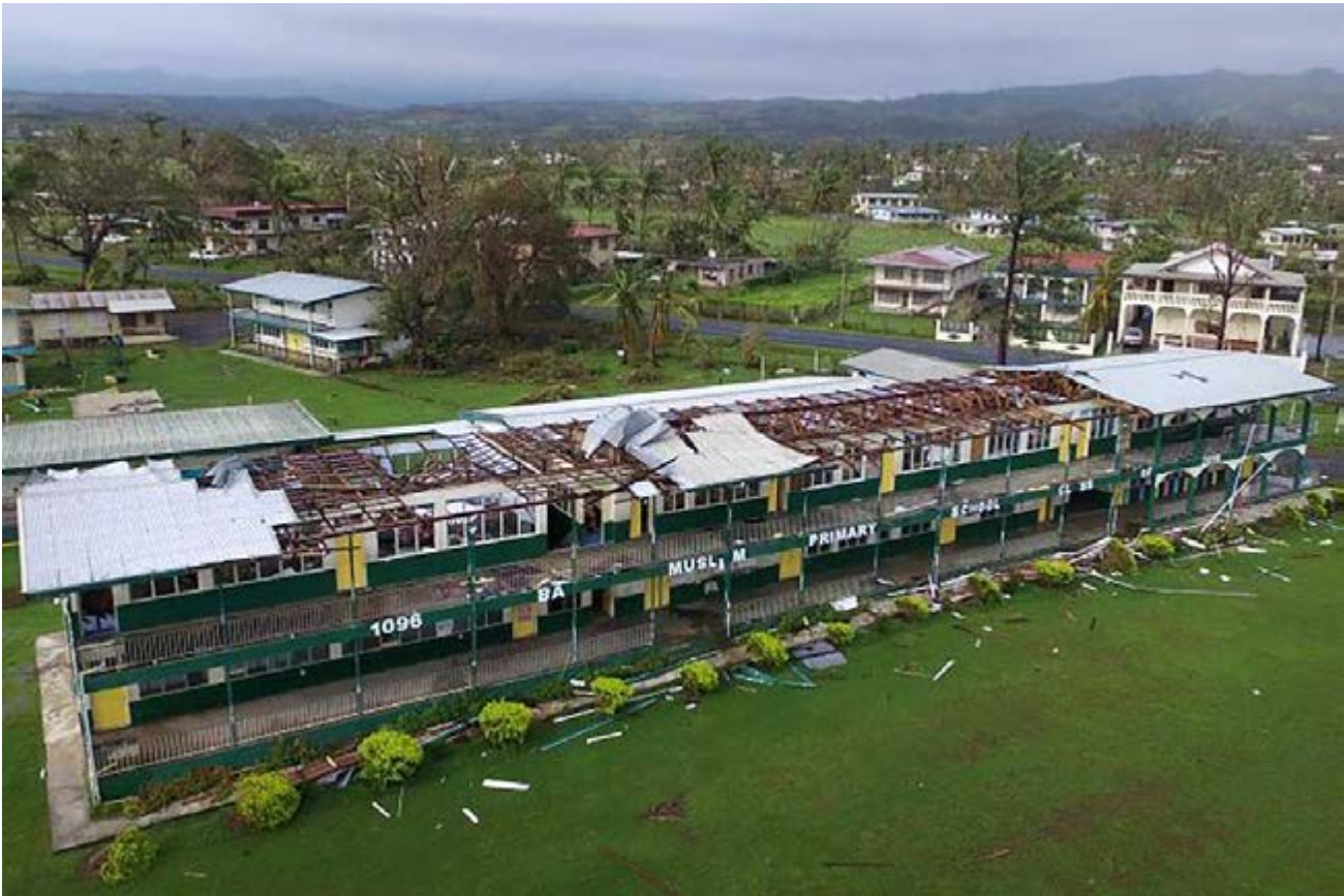
Muslim Primary School with roof torn off in the town of Ba near Lautoka
