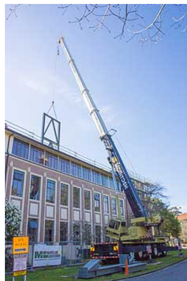
Sir Geoffrey Peren building during renovation
