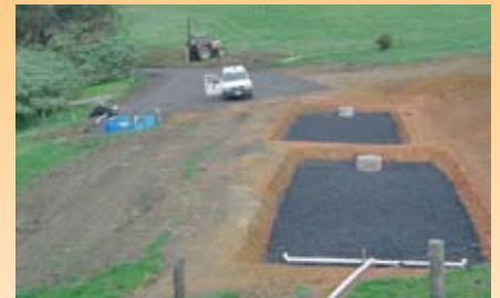
Above: Steelmaking slag in the laboratory and in situ in filter beds at a sewage treatment plant Below: Doctoral student Nicola Powell is working on how to make algae more phosphorus hungry and so a more potent means of cleaning phosphorus from water
