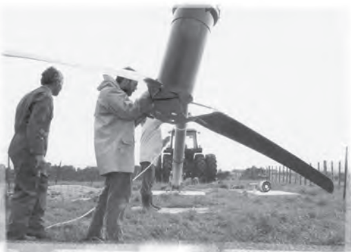
The wind turbine was installed on the Centre for Energy Research’s Renewable Energy testing site on campus in 1993, partly funded by the British High Commission. Research involves looking at ways to match local energy supply to meet remote rural community needs, thus reducing dependence on supplies through the national grid.
