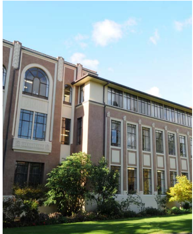
Sir Geoffrey Peren Building Manawatū Campus, Palmerston North
