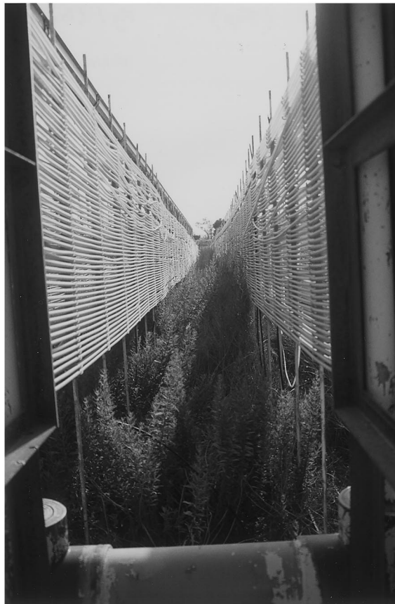
Fig. 1. A commercial horizontal tubular bioreactor facility that failed to perform to expectations and was abandoned. This facility was located in Cartagena, Spain and it was owned by Photobioreactors Ltd.
