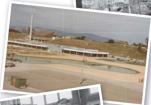
Vet clinic with lake and boiler house, 1968.
