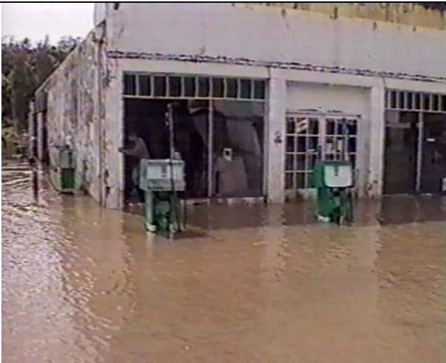
Figure 5 Garage flooded Source: TV3 News archives
