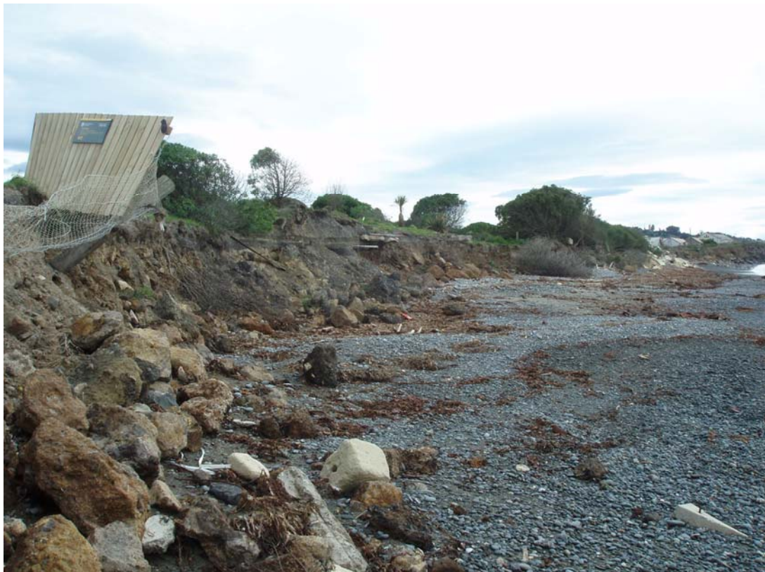
Figure 11: The Oamaru Creek Penguin Refuge. The upper photo shows the northern end of the refuge and the lower photo shows the southern end. The ends of the fence around the refuge have been truncated by the sea. The squared blocks of limestone are dumped masonry rubble which have had some effect in protecting the central part of the refuge from erosion. All of the currently exposed sea cliff at the refuge consists of rubble and reclamation materials. Photos 12 March 2009.
