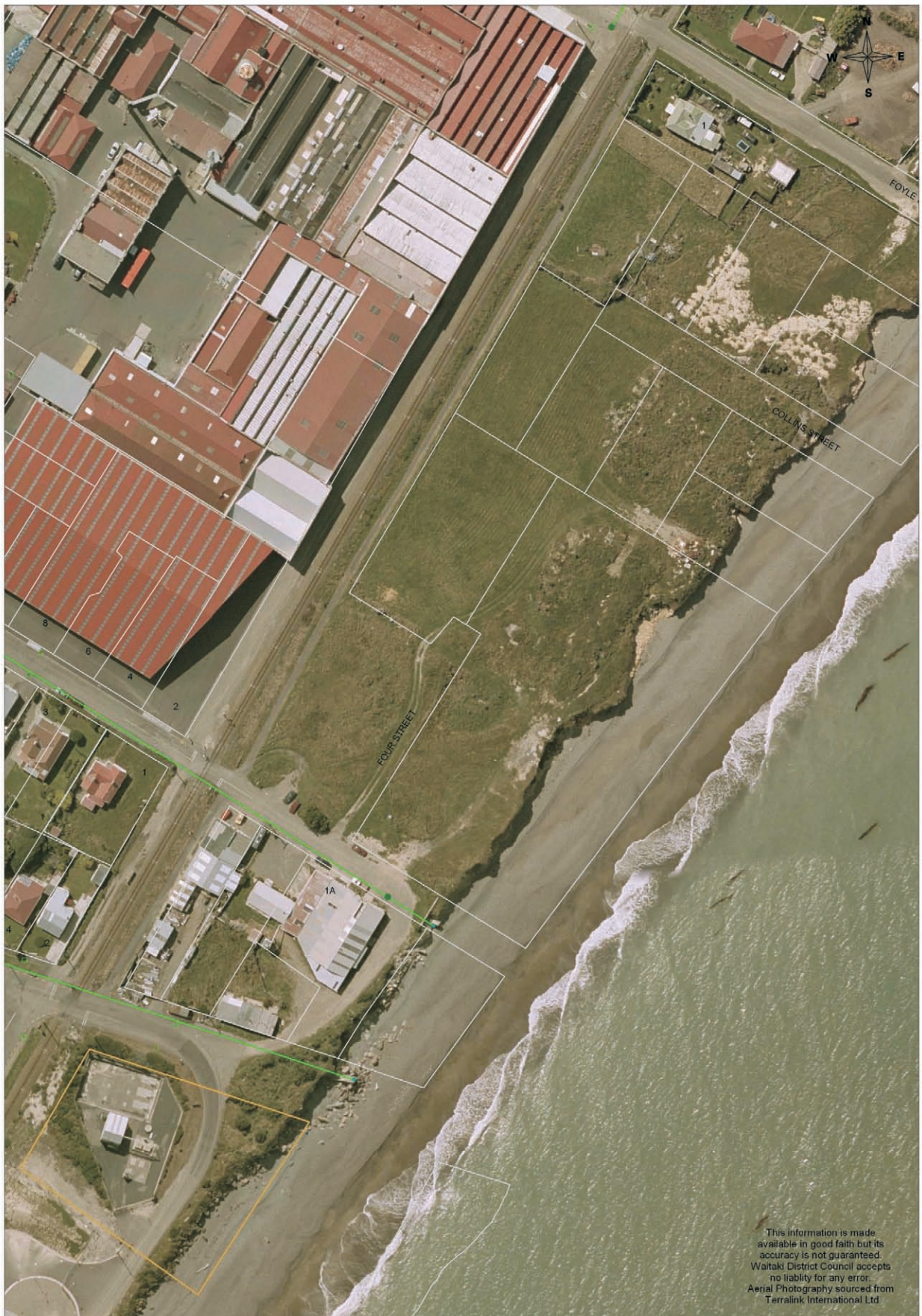
Figure 20: Cadastral data overlaid on a vertical airphoto dramatically illustrates the retreat of the coastline in northern Oamaru. The Firman joinery in Lower Weaver St is labelled as 1A. Stormwater pipes appear in green and a sewage pumping station in yellow. Note grey property boundary out to sea (lower centre). The coast has been eroded further since the photo was taken in 2005. This image was made available by Waitaki District Council, aerial photography sourced from Terralink International Ltd.
