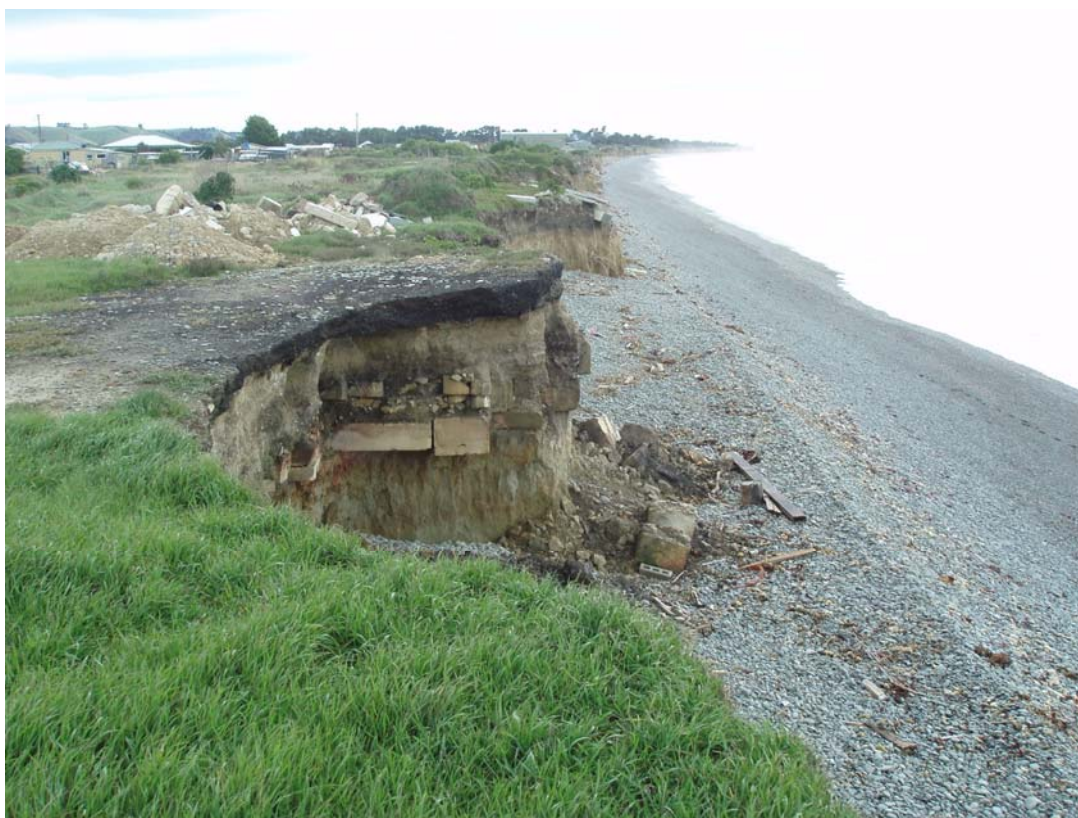
Figure 10: The present land surface, sea cliff and beach at Lower Weaver St, Oamaru, just north of the Firman joinery site (looking towards north). This area is visible in the background of Fig. 9 (upper). Squared blocks of limestone set into the top of the loess mark foundations of a former building, and modern deposits of spoil are also visible. Note storm beach (berm) well above present wave height, and more recent falls of material from the cliff onto this beach. Photo 12 March 2009.
