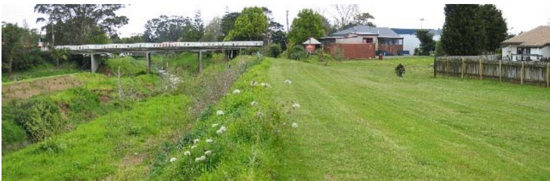
Figure 1. Panorama of stream, stop-bank and housing
