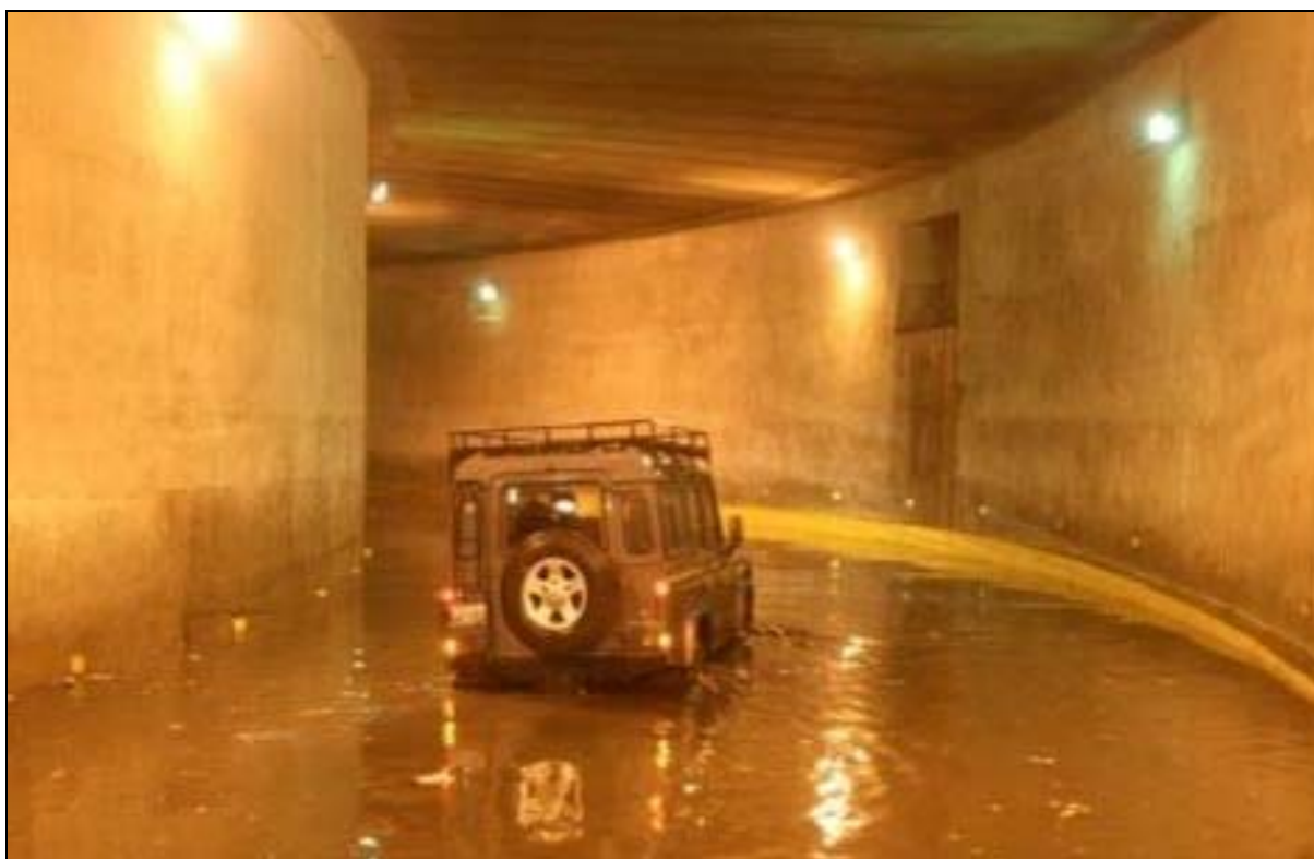
Figure 3.16 Flooded underpass, Guatemala City, early June 2010 (photo: Director of Works, Guatemala City municipality).
