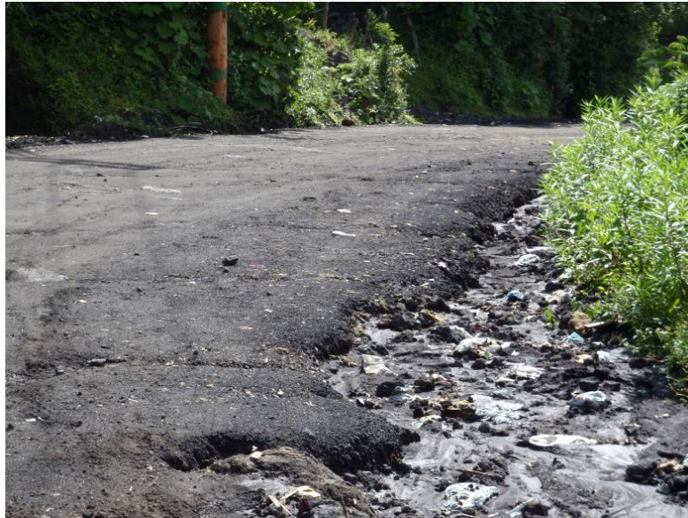
Figure 3.17 Road to San Francisco de Sales, showing compacted tephra road surface.
