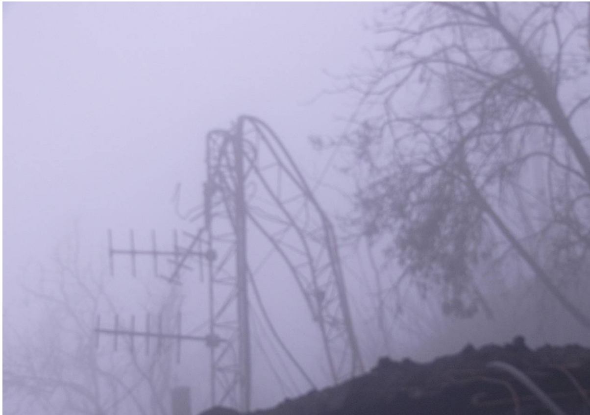
Figure 3.19 A radio communications tower on Cerro Chino that buckled from ballistic and block impacts (photo: Gustavo Chigna, INSIVUMEH).
