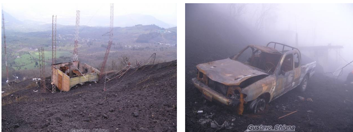
Figure 2.10 Ballistic clast damage to radio masts, building and vehicle in vicinity of Cerro Chino (photos: Gustavo Chigna, INSIVUMEH).
