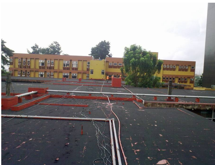
Figure 3.10 Roof of hospital B covered in tephra.
