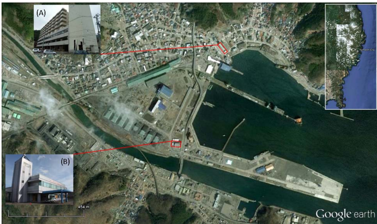
Figure 34 Designated evacuation locations in Kamaishi City. An estimated 50 people evacuated to this apartment block (A) and government offices (B). The entire area shown was inundated; inundation depth was 8 m in the vicinity of building (A).
