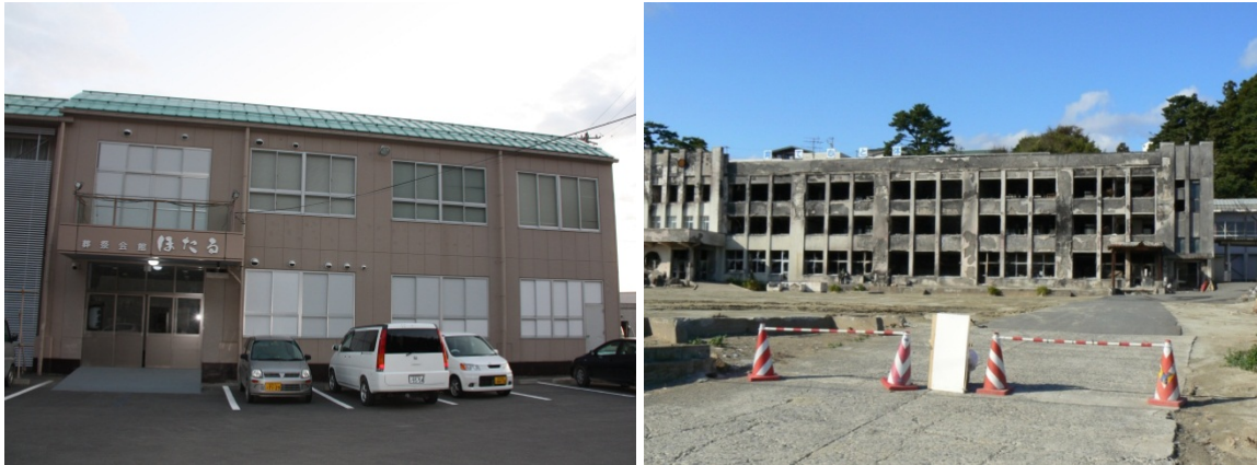
Figure 62 The Hotaru funeral facility. This is an unlikely vertical evacuation facility given the lack of obvious roof space or external access, but successfully provided refuge on March 11 th .
