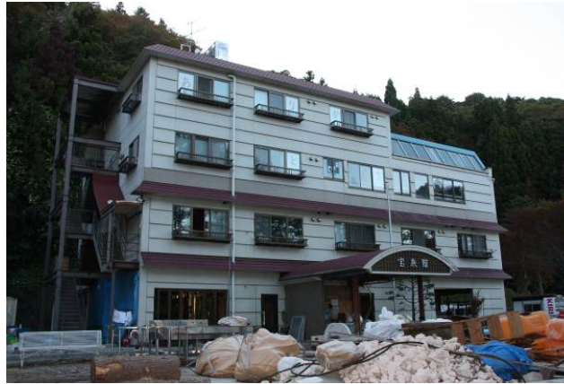
Figure 37 The Hotel Horaikan at Unosumai, Kamaishi City, with official signage displayed at the 3 rd floor and very little external damage. The hotel was inundated to the ceiling of the 2 nd storey
