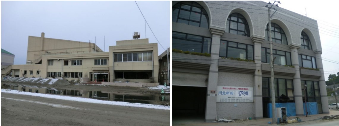
Figure 52 Kesennuma central community centre, where 450 people took refuge when they evacuated nearby buildings
