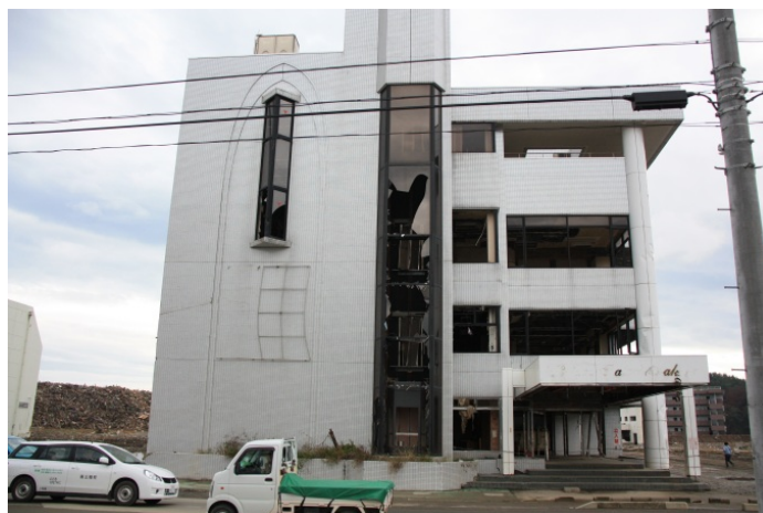
Figure 56 The Takano Kaikan building 160 m inland of the Matsubara apartment block. Little damage aside from glazing was observed here, despite heavy damage and collapse of RC buildings immediately seaward.
