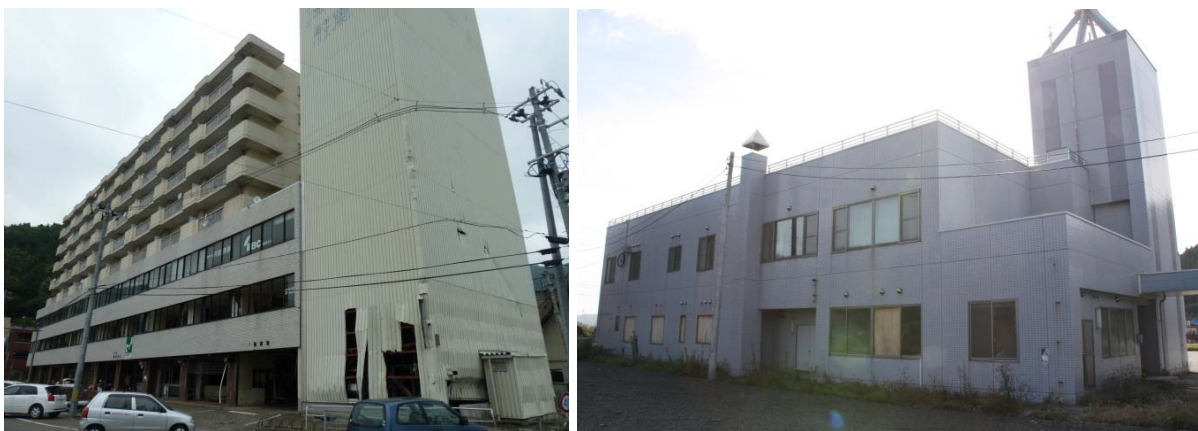
Figure 35 Apartment block in Kamaishi City, which was inundated to the 3 rd storey
