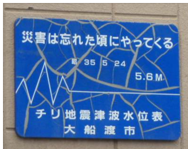
Figure 30 Tsunami height marker on a building wall in Ōfunato City, indicating the maximum inundation height at this point during the Chile tsunami on May 24 th 1960. Photograph courtesy of EEFIT.
