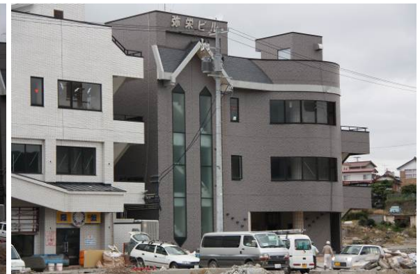
Figure 41 Yasuka private commercial and apartment block number 1 shows very little exterior damage.
