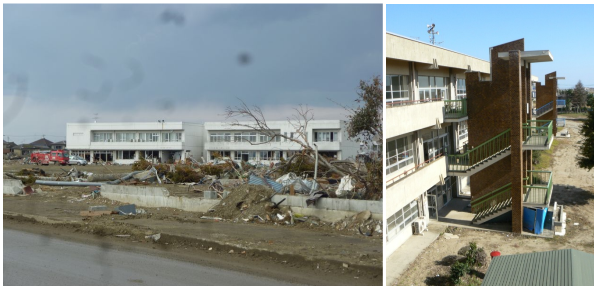
Figure 65 The Yuriage Community Centre was inundated to the 2 nd storey but 43 people survived in the building.
