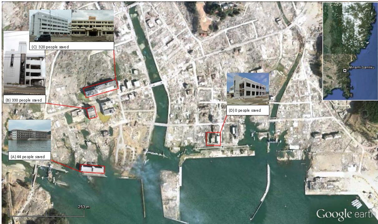
Figure 54 Locations of designated tsunami evacuation buildings in Minami-Sanriku Town: (A) Matsubara apartments; (B) Takano Kaikan building; (C) Shizugawa Hospital; (D) Fisheries Co-operative. Significant scour can be seen where seawater is encroaching around building (A) and to the east of building (D).
