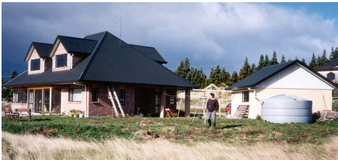
Figure 1 Household rainwater collection and storage system (M. Rosenberg photo).
