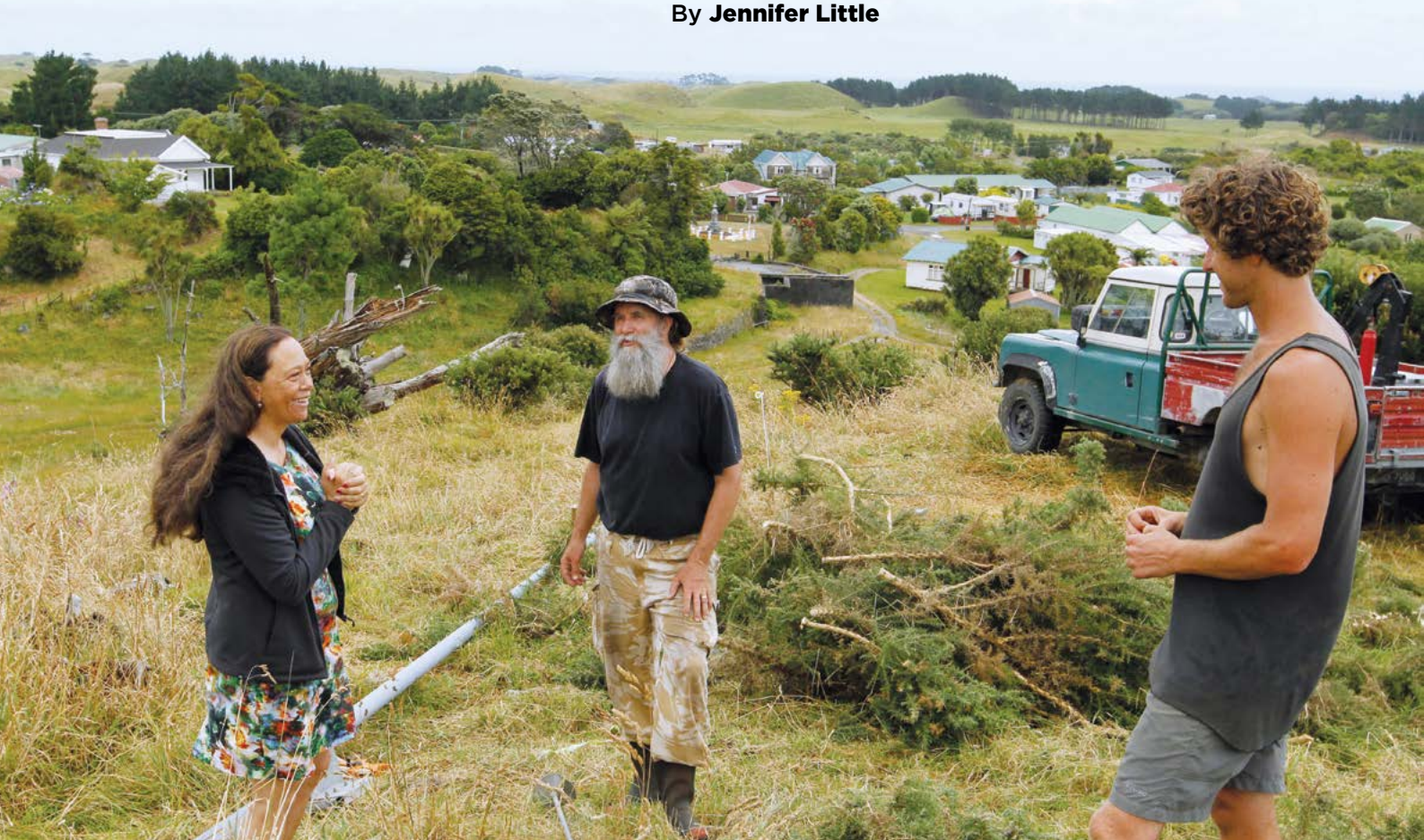
Amokura Panoho, Dr Phil Murray and masterate student Josh Curd at Parihaka as they begin to erect a tower to hold equipment for measuring wind and sunshine.
