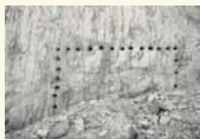
Drill line, new underground dwelling, Coober Pedy, Australia 2003
