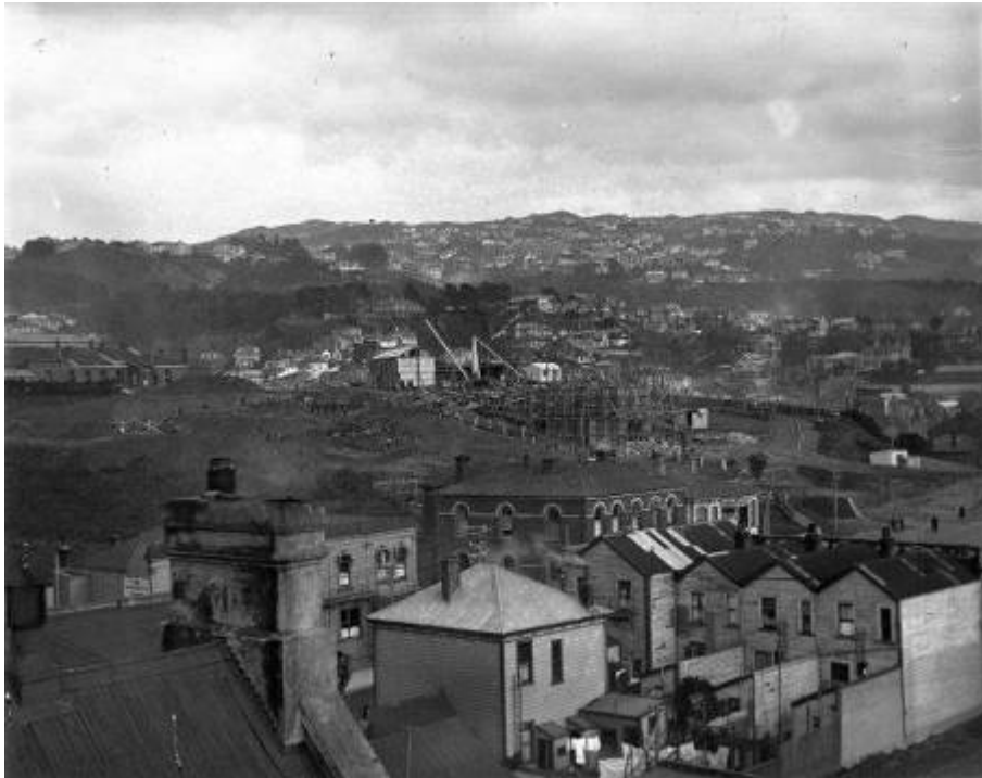
Carillon under construction. Negatives of the Evening Post newspaper. Ref: 1/2-090208-G. Alexander Turnbull Library, Wellington, New Zealand. http://natlib.govt.nz/records/22912964
