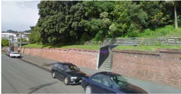
Tasman Street retaining wall – centre
