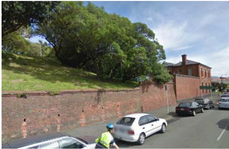
Tasman Street retaining wall – northern end.
