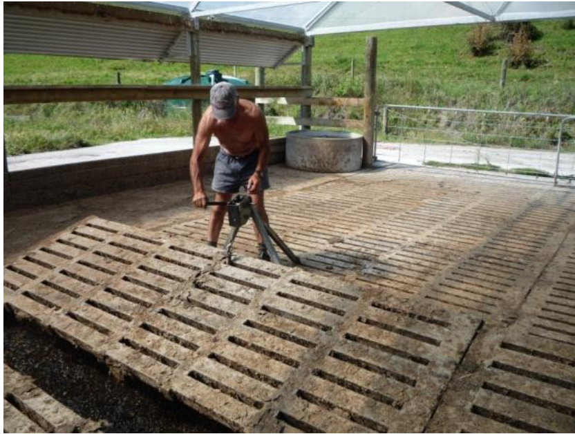
Plate 1: Tripod assembly easily winches slat allowing access to bunker manure.
