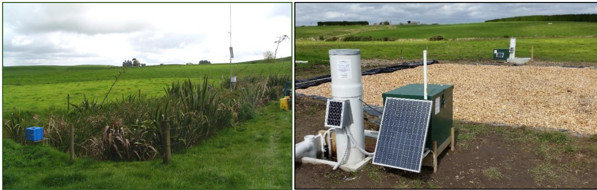
Figure 1: Current mitigation systems for agricultural drainage treatment: constructed wetland, at Toenepi Waikato and woodchip bioreactor at Waituna, Southland (C. Tanner).
