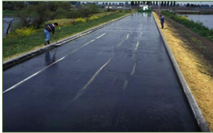
Figure 2: Filamentous algal nutrient scrubber at field scale in California, USA. (Rupert Craggs)
